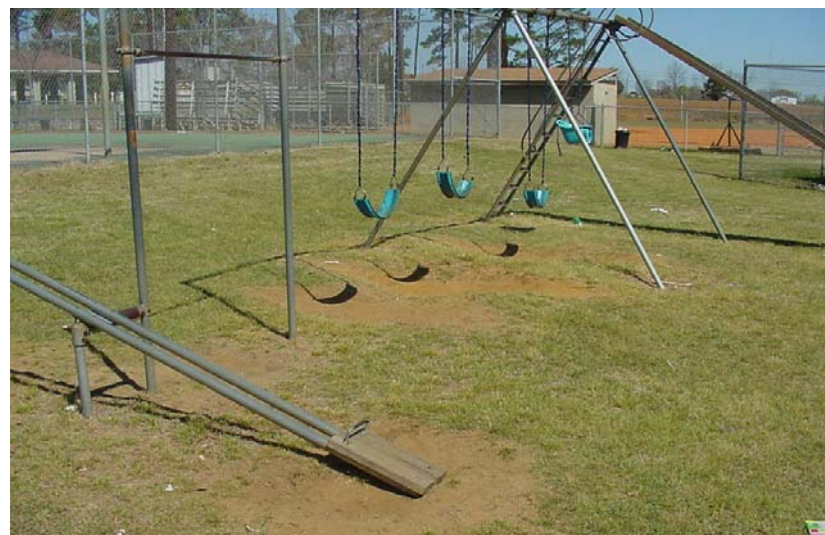
This playground doesn't use any protective surfacing in the event of a fall.
