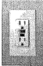
Outlet type GFCI
